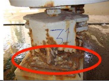
Completely rusted Spring Hangers after years of services.
