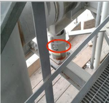
Improper installation – blocking not removed properly.
