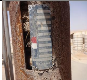
Corrosion worsened by painting rather than by using HDG.
