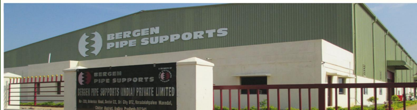
BERGEN PIPE SUPPORTS (India)
