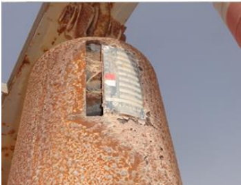
Corrosion worsened by painting rather than by using HDG.
