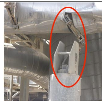
Stress Analysis not done properly, huge misalignment causing breakage.
