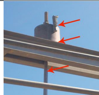
Blocking of Spring Hanger was done incorrectly. Hanger is misaligned due to the absence of a base plate. Hanger Rod is bent due to misalignment of Spring Hanger.
